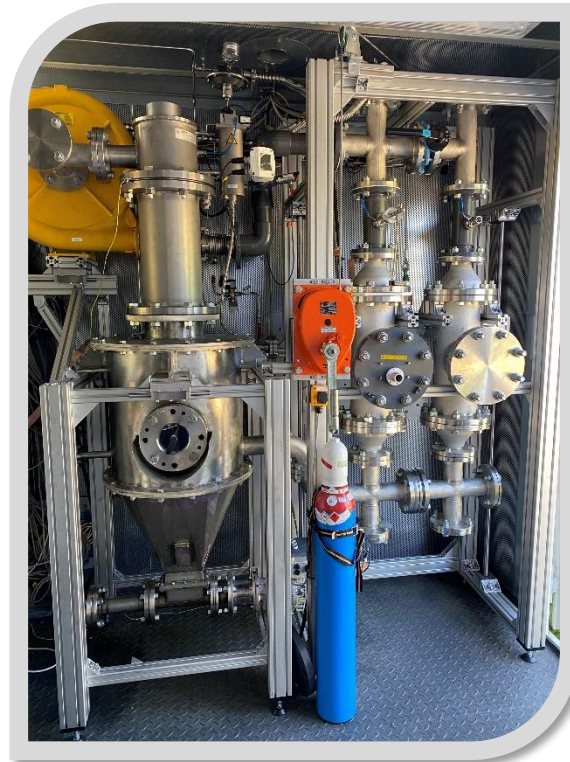
Hotel MOA H 2 -blending heating boilers for CO 2 reduction
