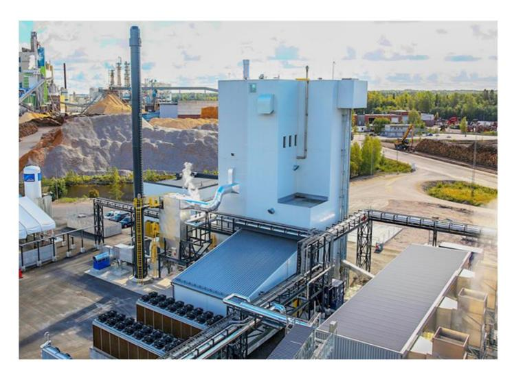
Commercial production of Pyrolysis oil from saw dust for advanced biofuels
