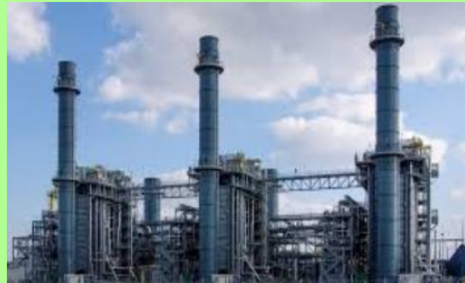
Natural Gas Power Station
