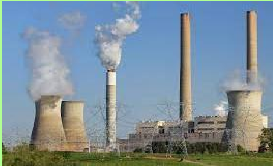
Thermal Power Station
