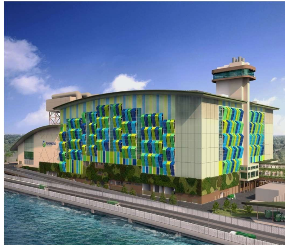
WtE plant in Singapore
